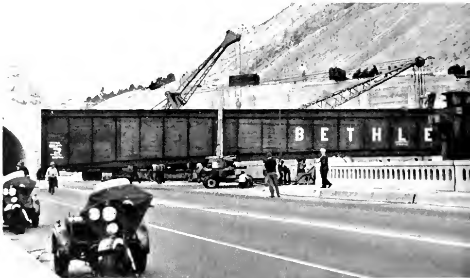
Moving this 146 foot girder weighing 82 tons closed city streets three hours
